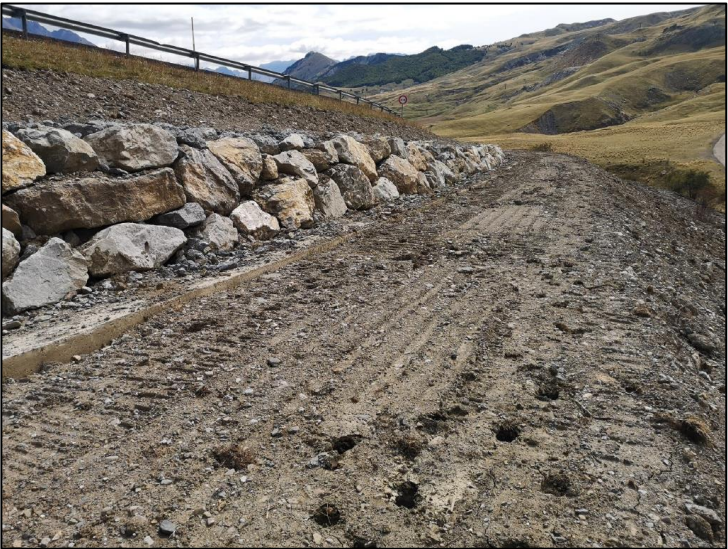
Installation securing a road from landslides
